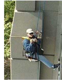
Investigation of Curtain Wall Using Roped Access Building Complex Englewood, Colorado
