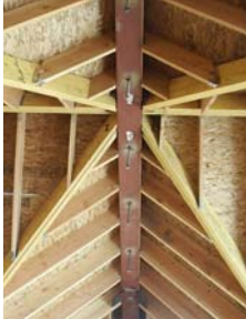
Structural Evaluation of Wood Framing Top of Mill Condominiums Aspen, Colorado
