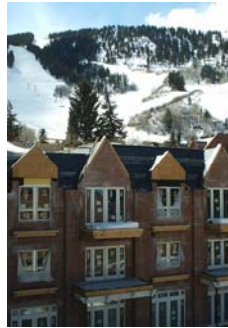
Snow Country Roofing Evaluation Hyatt Grand Aspen Hotel Aspen, Colorado
