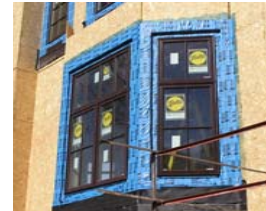
Window Installation Mock-Up Broadmoor Brownstones Colorado Springs, Colorado
